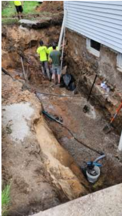
North Wall Excavation
