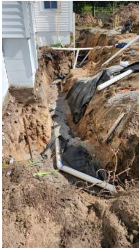
East Wall Excavation
